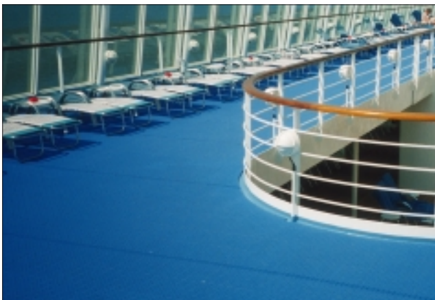
Installation on board NORWEGIAN SKY
