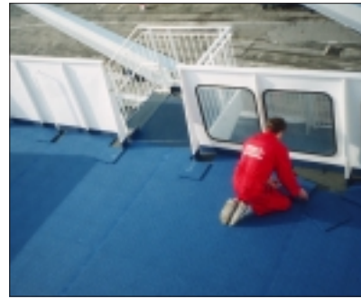
Easy to install, NO fastening, adhesives or special tools are needed. The tiles lie on top of the subfloor.
